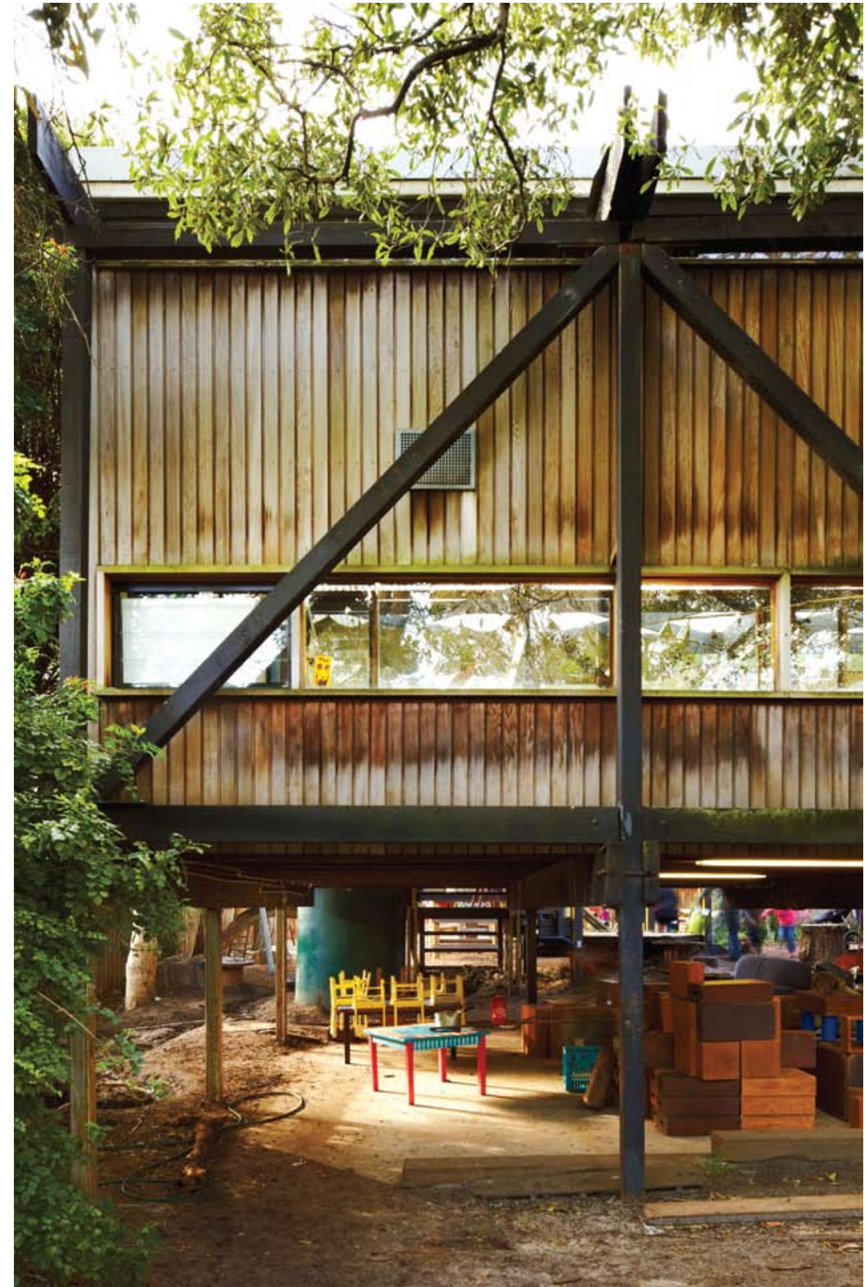
Undercrofts provide extra space in what is a surprisingly small site.
