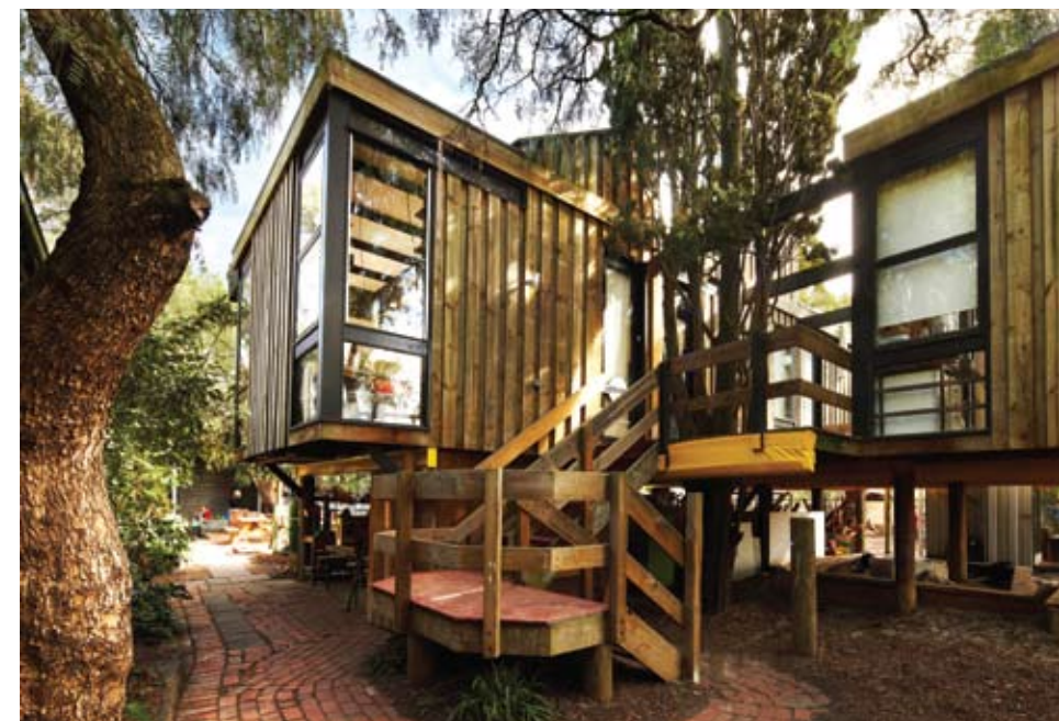
The 'tree house', constructed in 1965 – two elevated classrooms separated by a timber deck and an Italian Cypress.
